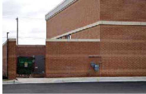
This service area enclosure is integrated with the building and appropriately located to the rear of the lot
